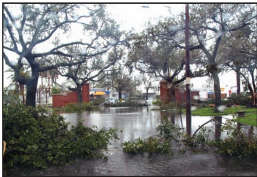
The campus of the New Orleans Baptist Theological Seminary sustained heavy damage from Hurricane Katrina and from the subsequent flooding when the levees broke.
