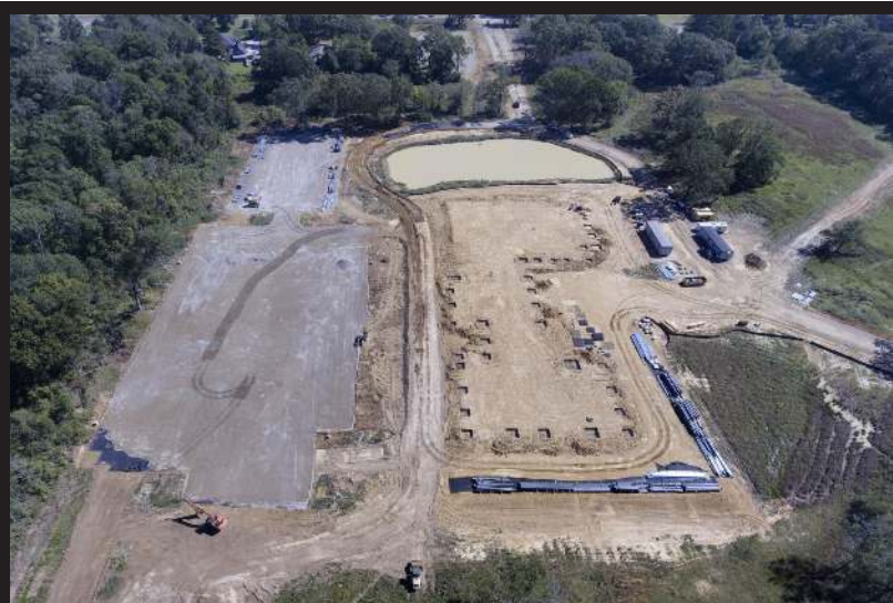
First Baptist Church Denham Springs—Under Construction
